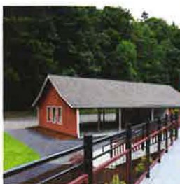
BEACH PARK PICNIC SHELTER
